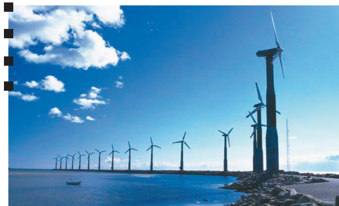
Ebeltoft wind farm, Denmark.
