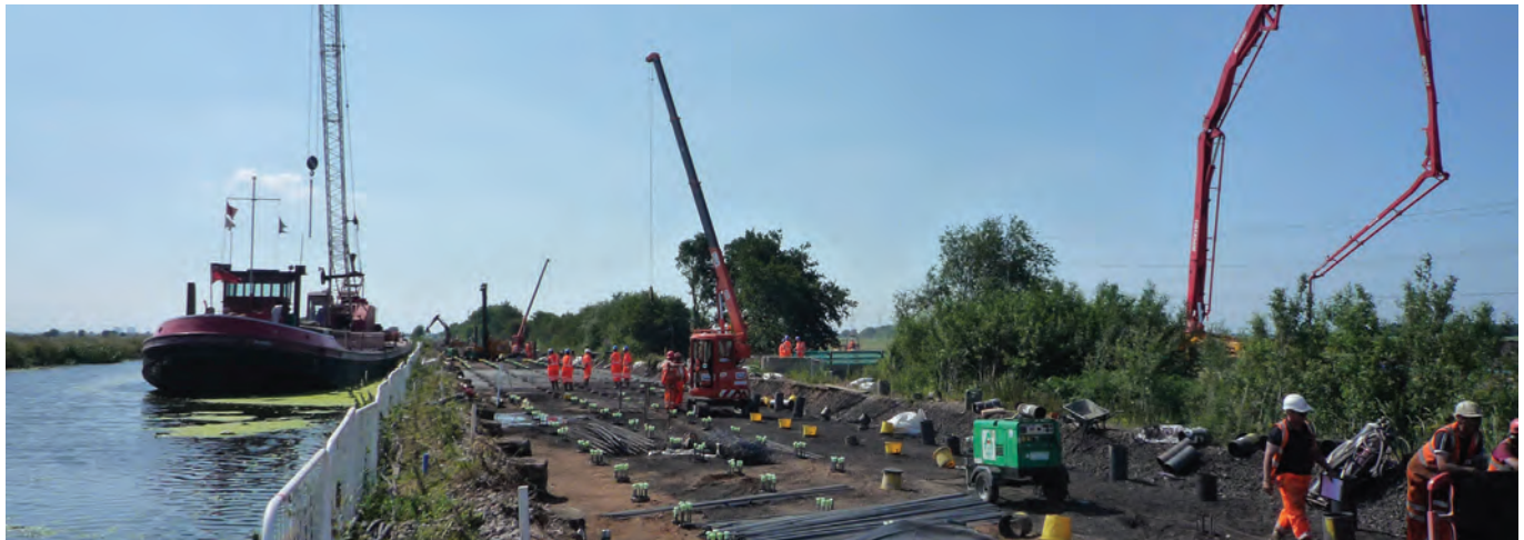
The upgrade works took just 11 weeks to complete
